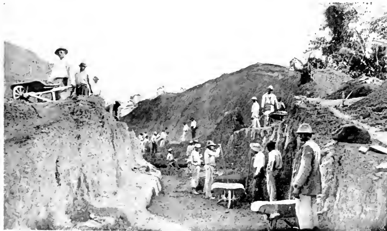
A CUT ON THE VIENTO FRIO BRANCH.
